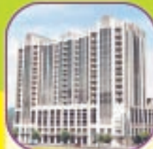
10 Paramount on Lake Eola 16-story, mixed-use residential tower, including a Publix grocery. Construction starts: 1st quarter 2006.
