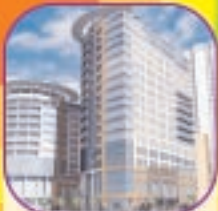
7 Premiere Trade Plaza 13-story office tower, 17-story office tower, 27-story condo tower called the Solaire, retail space and a 12-screen movie theater. Under construction, completion 4th quarter 2006.
